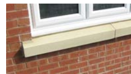
Cast stone cills and lintels
