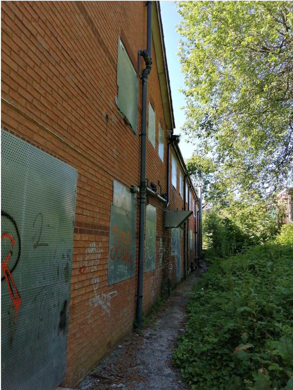
Photo 4: The eastern elevation of the existing building
