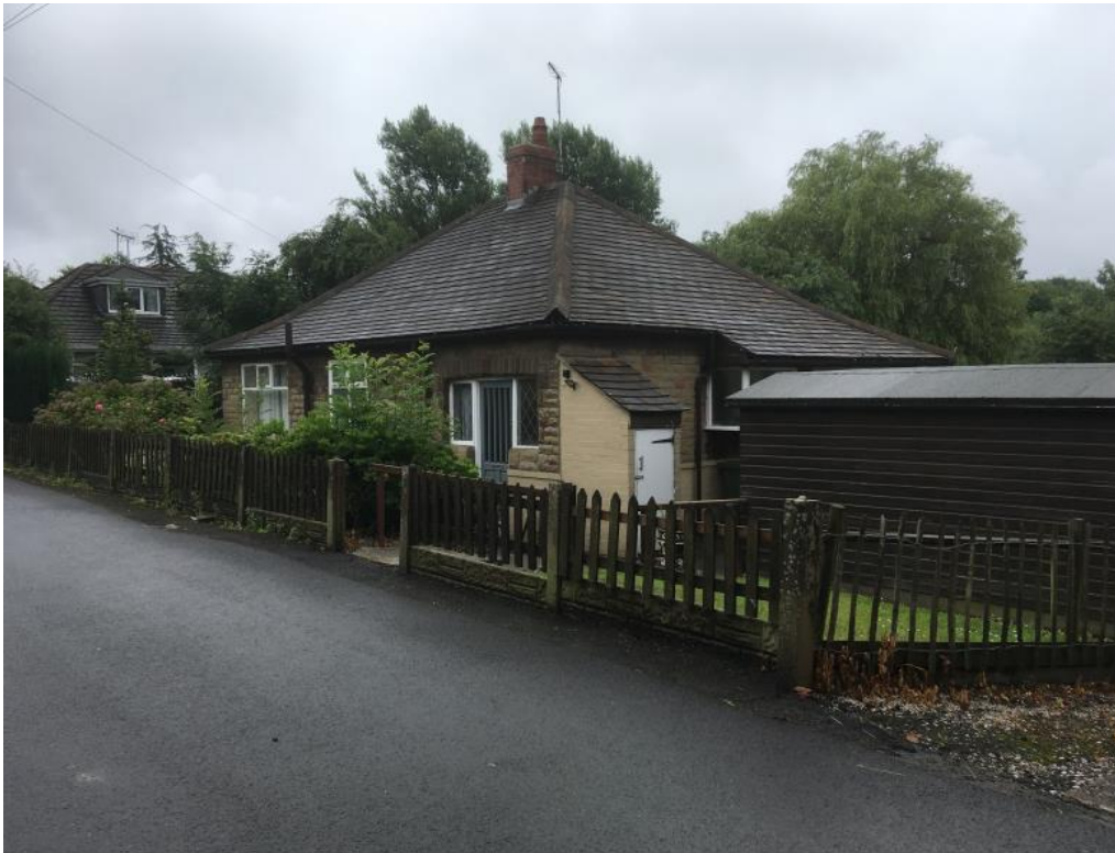
Photo 2: No.10 Slate Lane (to be demolished)
