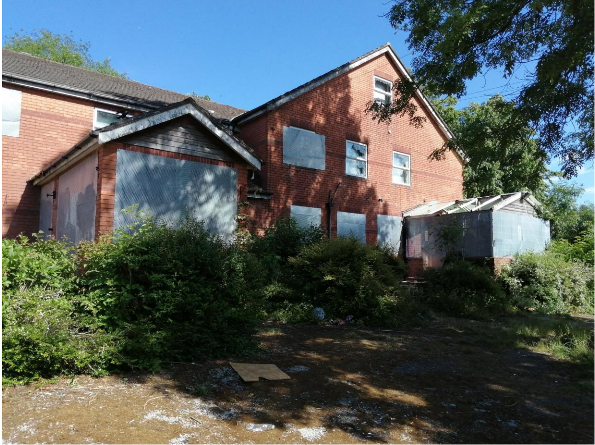
Photo 2: The existing building viewed from the west
