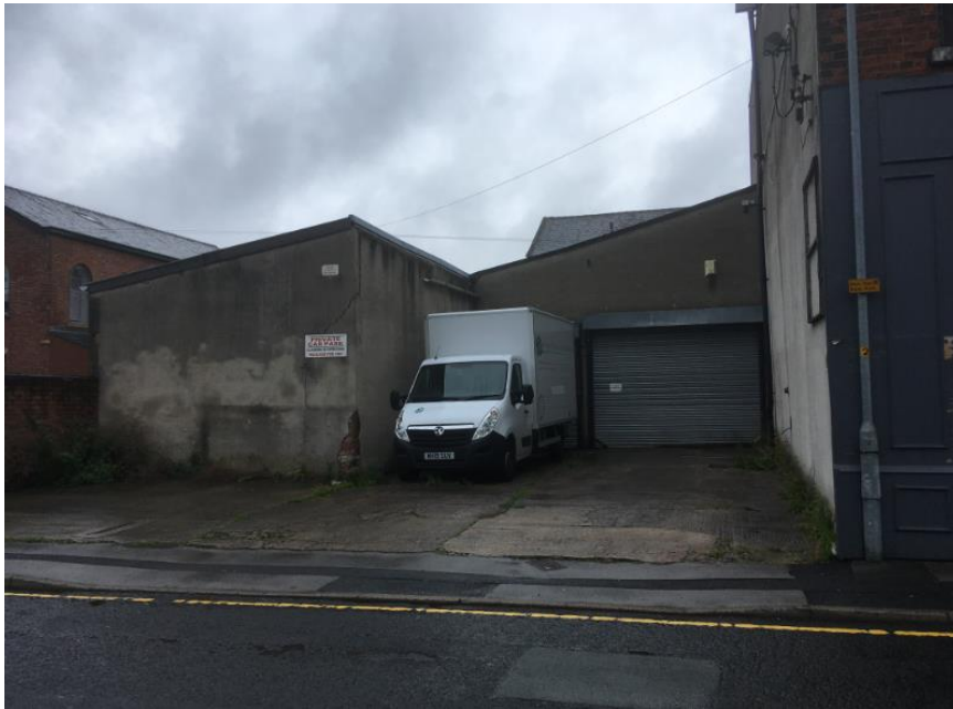
Photo 5: Lean-to to be demolished.
