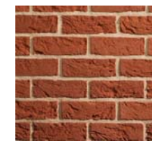
Red brick plinth
