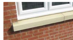
Cast stone cills and lintels
