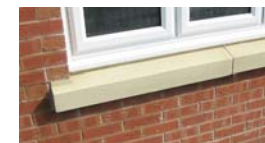
Cast stone cills and lintels
